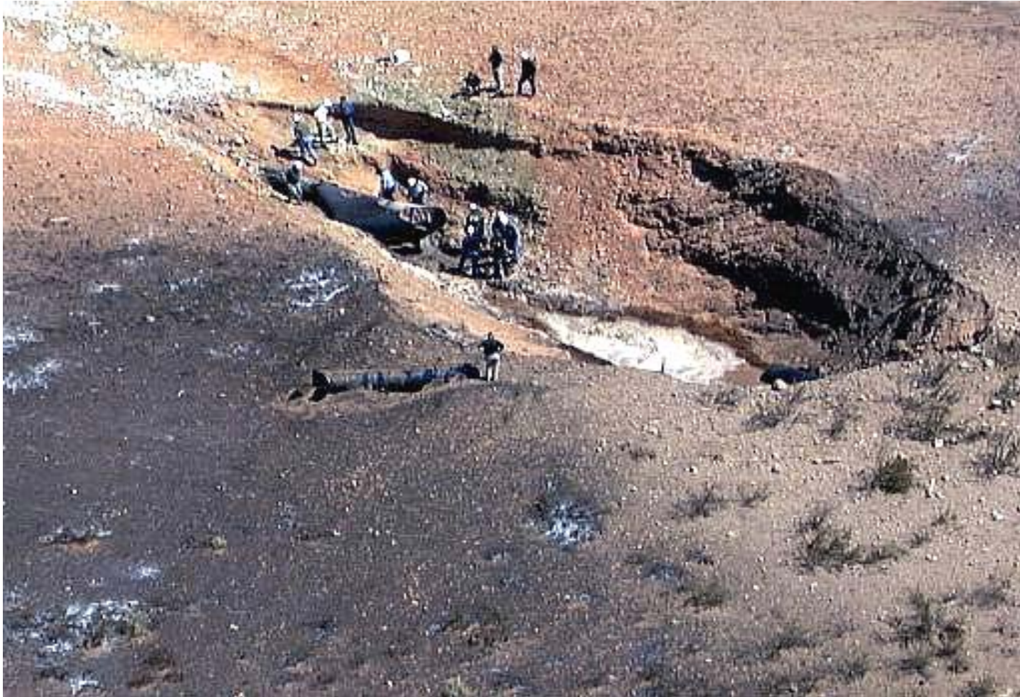
Carlsbad pipeline explosion, New Mexico USA in August 2000
